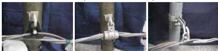
French System Insulated Phase Conductors & Insulated Messenger Dead End Clamp
