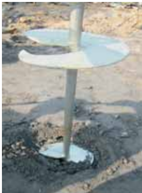
Beginning of the application test by screwing in the anchor
