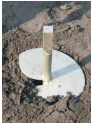
Application Test for Helix Anchor has screwed in
