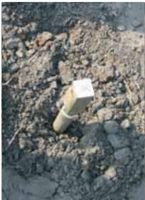
Triple Helix Anchor now Fully Installed
